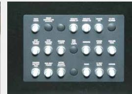
Resettable circuit breakers eliminate fuses
